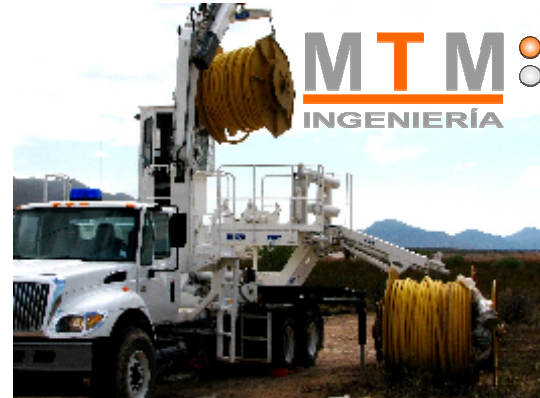
Drums in operation
